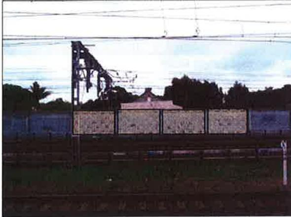
**OR REMOVE AT LEAST TWO HORIZONTAL PANELS & REPLACE WITH SINGLE SHEET
